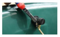
4. Where necessary bend the lever arm to adjust the water level. This can be done by removing the lever arm assembly. Remove R-pin and slide the pivot pin with a pair of pliers then slide it out.
