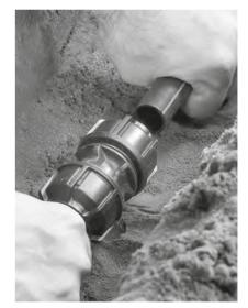
**6. Disassembly** To disassemble the fitting simply loosen the nut using a wrench until 2 threads are showing. Pipe will be released and can simply be pulled out of the fitting.
