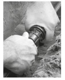
**4. Nut Tightening** The nut should be tightened by hand and then firmly with a wrench. Tighten the nut all the way to the flange on the body of the fitting.
