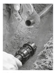
I. Cut Pipe Square Cut the pipe square. There is no need to prepare the pipe end. Chamfering or lubrication is not required.
