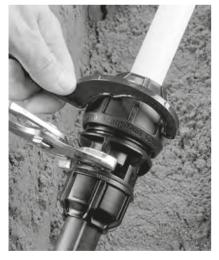
**4. Nut Tightening** Tighten nut firmly with a wrench. Nut will not butt against the body flange when the pipe size is at the top end of the fitting tolerance.
