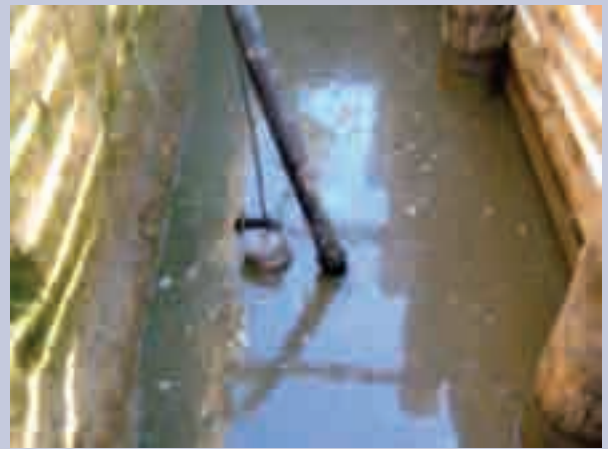
Weeping Wall settling bed for dairy effluent
