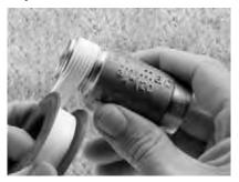
Apply PTFE tape or approved sealant to the thread ensuring a sufficient amount is applied to guarantee a watertight seal.
