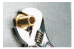
Refit the backnut and tighten with a spanner. The valve body\*\* can be held in place with a spanner, multi-grips or equivalent.
