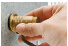
2. Where using the stem sleeve to fit the valve into ¾" holes, ensure it is properly located on the valve side of the installation to prevent the valve moving.
