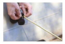
Where necessary bend the lever to adjust the water level. This can bedone by removing the circlip, sliding out the pivot pin and removing the
