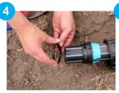
Slide the components onto the pipe, first the nut, then the split ring and collet followed by the O-ring.
