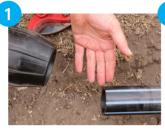
Cut the pipe square. There is no need to chamfer or lubricate the pipe.
