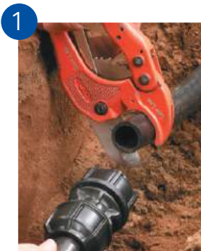
Cut the pipe square, there is no need to chamfer or lubricate the pipe.
